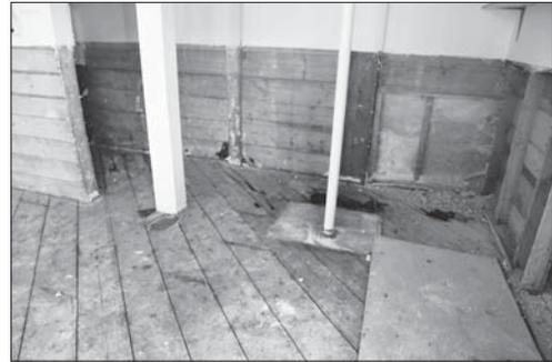
When 16 inches of water filled the basement dance studio, it caused extensive damage, and revealed pre-existing rotting and damage underneath the floor of the building.
