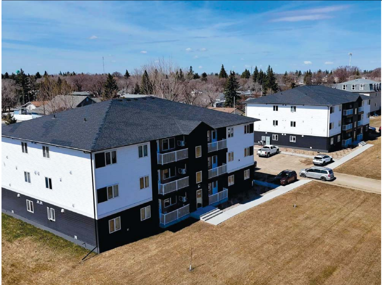
These two 12-unit apartment buildings were completed by Keller Developments under the housing accelerator program.
