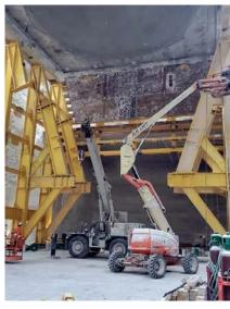
North coarse ore bin steel installation at K3.
