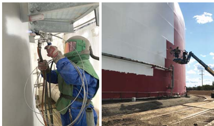
Above left: DC17 painters specialize in applying a variety of protective coatings as seen here with a member applying thermal spray aluminum metalizing Above right: DC17 Painters hard at work painting a storage tank
