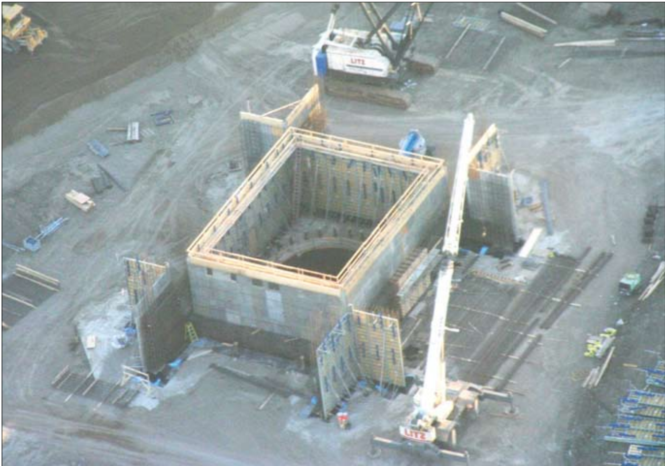
The base of the new headframe, which will rise 192 feet over 10 days in November.
