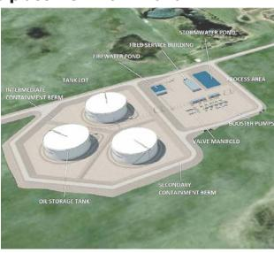
As part of its quarterly update on Energy East filed with the National Energy Board on Sept. 30, TransCanada released these updated proposed layouts of the pump station and tank farm to be added at the site of the Moosomin Compressor Station, which is located northeast of town. The tank terminal would include three 350,000 barrel tanks for a total capacity of 1,050,000 barrels of oil.
