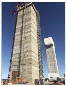
The continuous pour on the south headframe at K3, part of the \$3 billion expansion of Mosaic Esterhazy's K3, was completed on September 4 three days ahead of schedule. At 380 feet, the north headframe at right in the photo is the tallest structure in Saskatchewan. Crushrite Concrete provided the concrete for the pour. the south headframe. The slipform went up in a continuous pour, rising at 6.5 inches an hour for 24 days.
