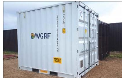
A shipping container converted to a sample dryer has increased the ECRF's capacity to complete more trials and dry grains and forages in a timely manner.
