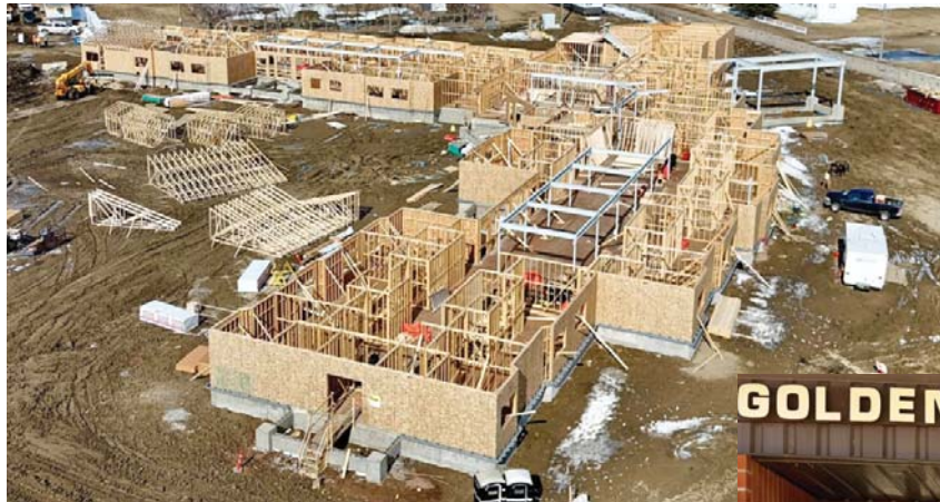
The new long-term care facility under construction at Grenfell.
